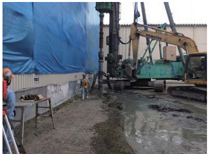
PHC杭削孔
