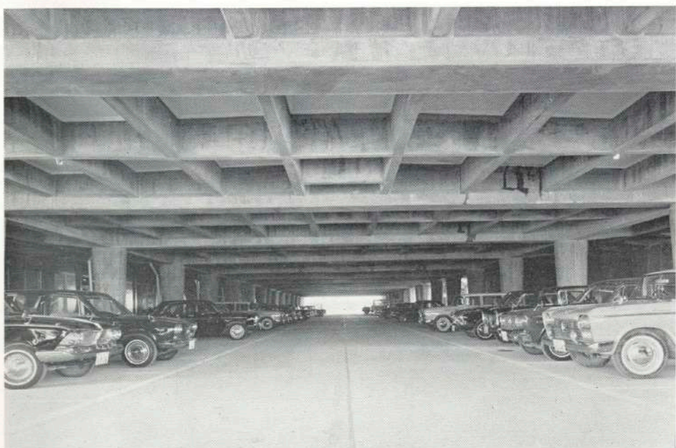
事務棟1階駐車場 Office wing, 1st floor parking
