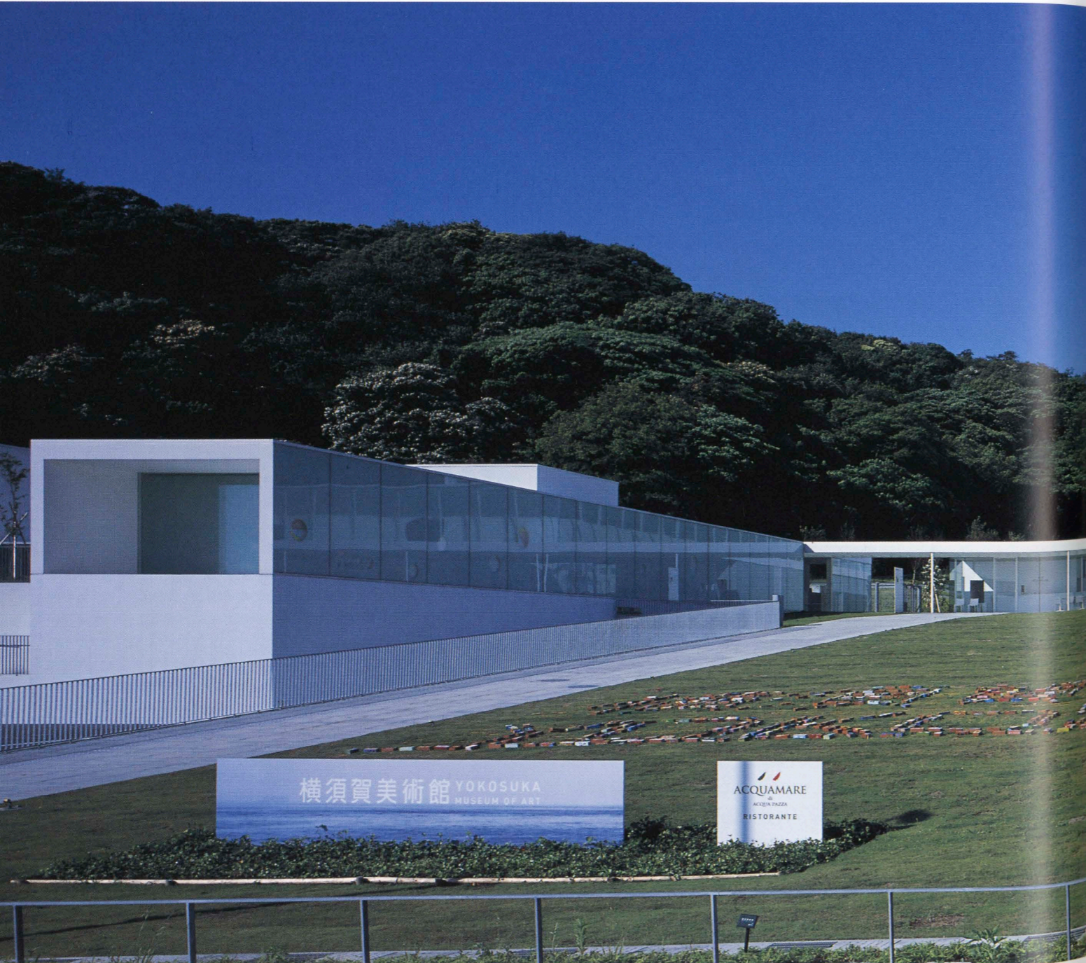
北東(海側)より見る全景 General view from the northeast (sea side).
