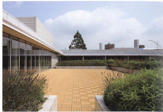
南館3階テラス View of the terrace on the third floor of the south building.
