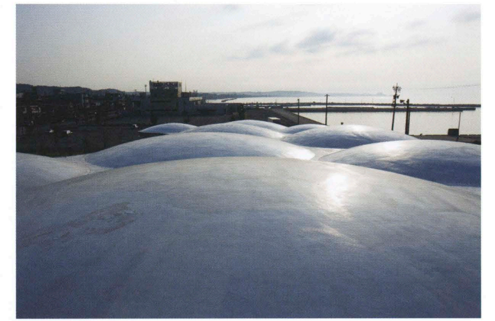
屋根より北側を見る North view from the roof.
