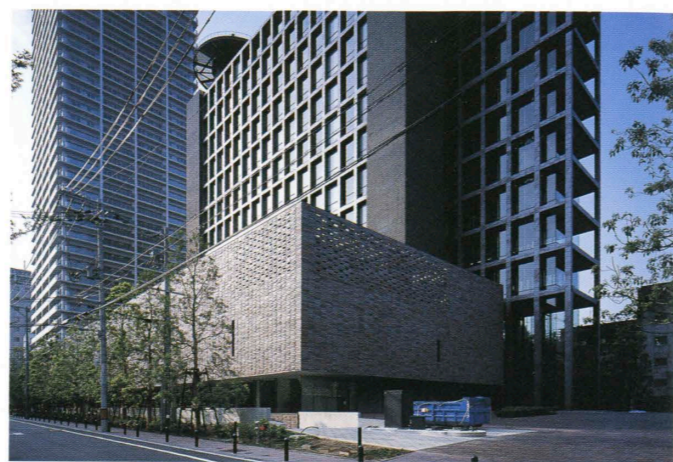
東側外観 Exterior view of east side.
