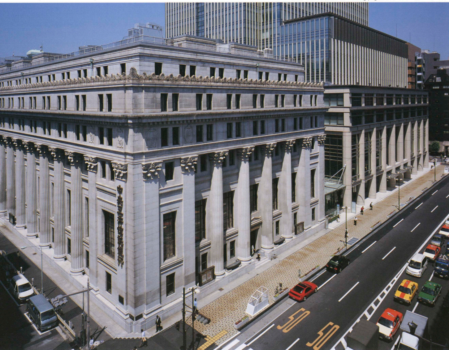
南東より低層部を見る View of the lower level from the southeast.
