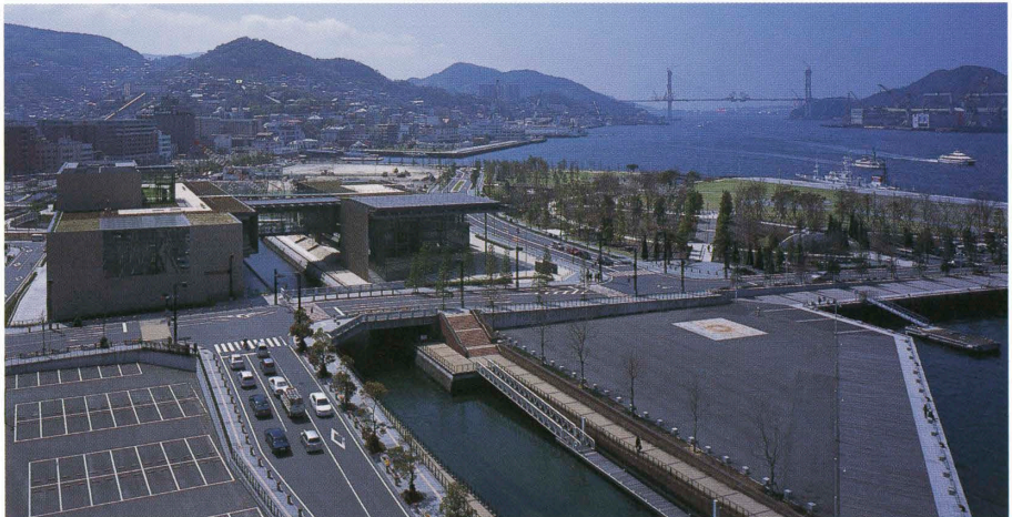
北側全景 General view from the north.
