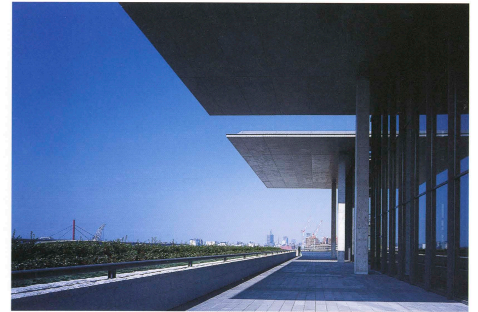
庇下の基壇部 Space under the eaves on the second floor.
