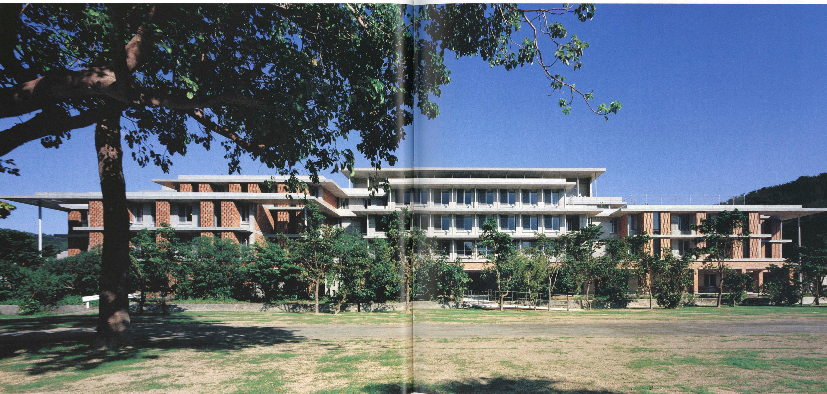
南側外観 South view.
