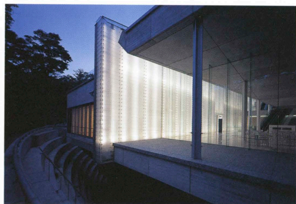
地下2階の光壁 Lighting wall on the second basement floor.
