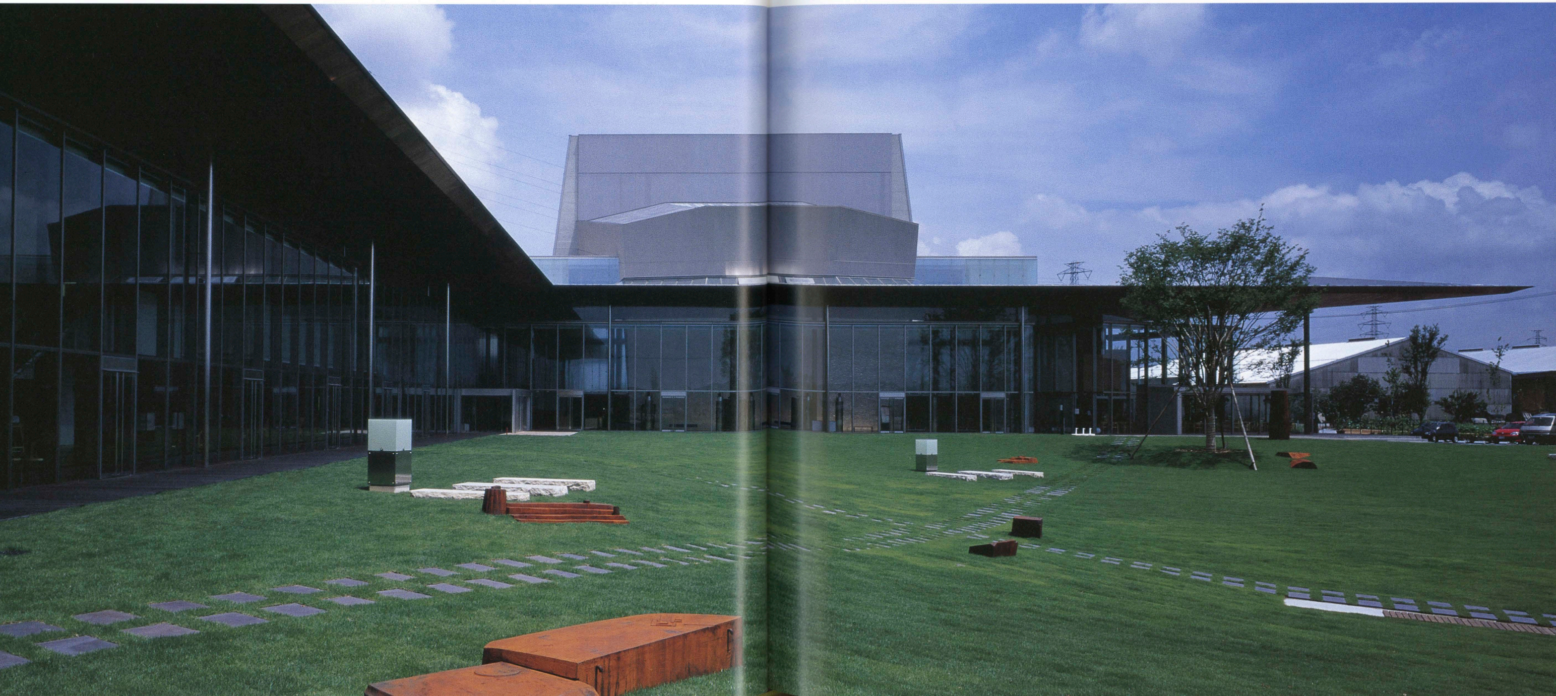
南側より見る View from the south.
