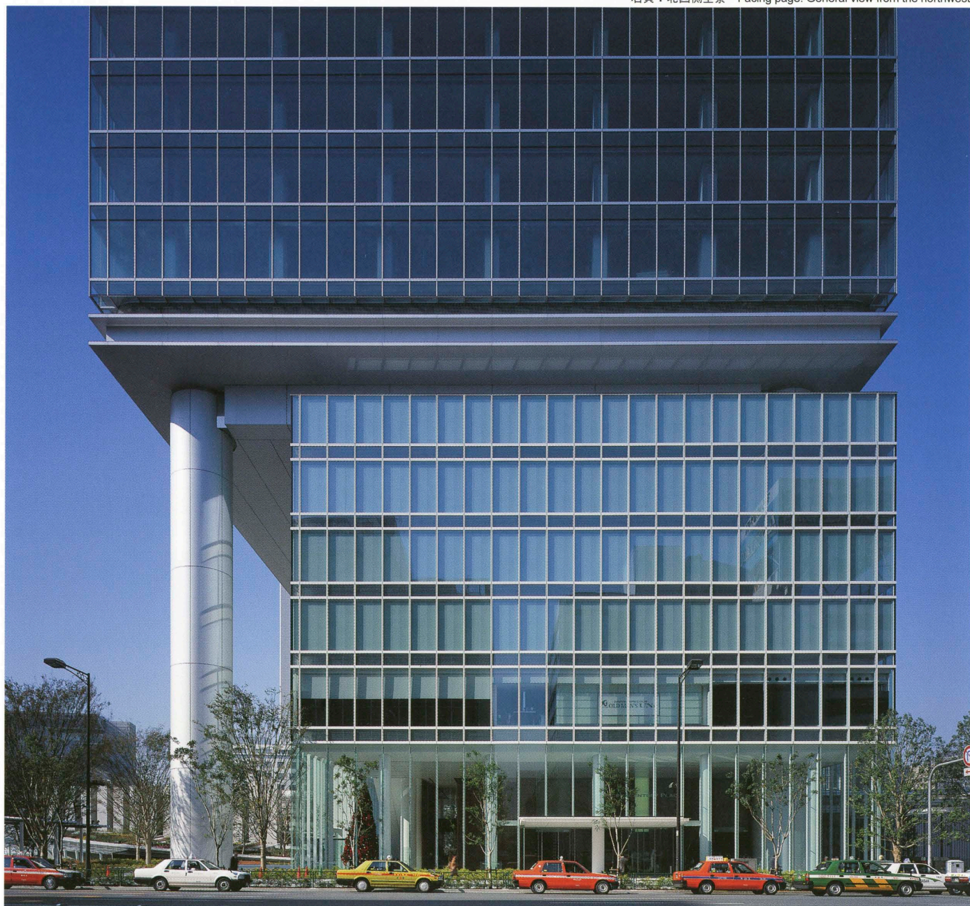
東側足元を見る スーパーコラムの直径は3,400mm View of the foot of the building. Diameter of the super-column: 3,400mm.
