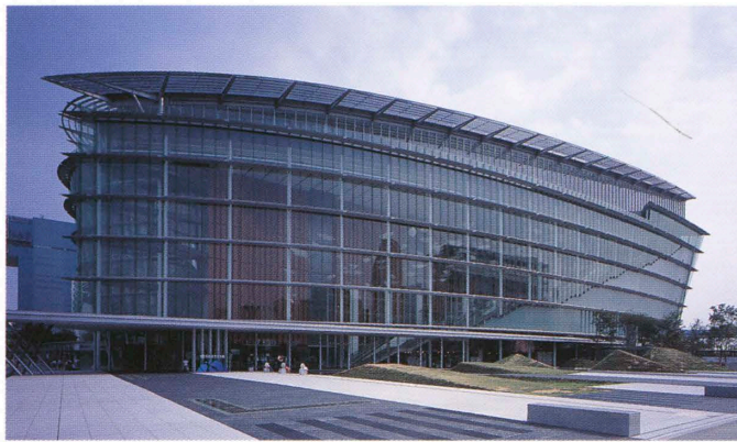
北側全景 General view from the north.
