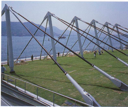
屋上広場 Grass-covered plaza on the roof.
