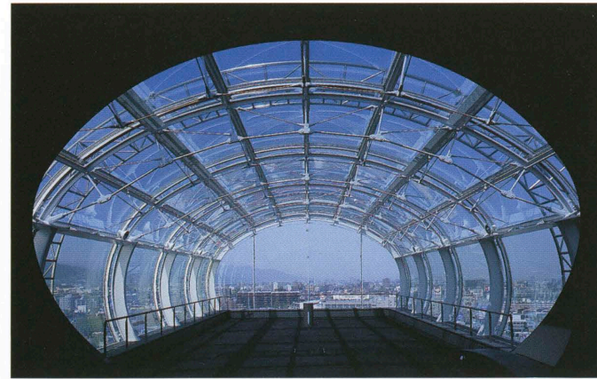
展望台内部 Interior of the observatory.
