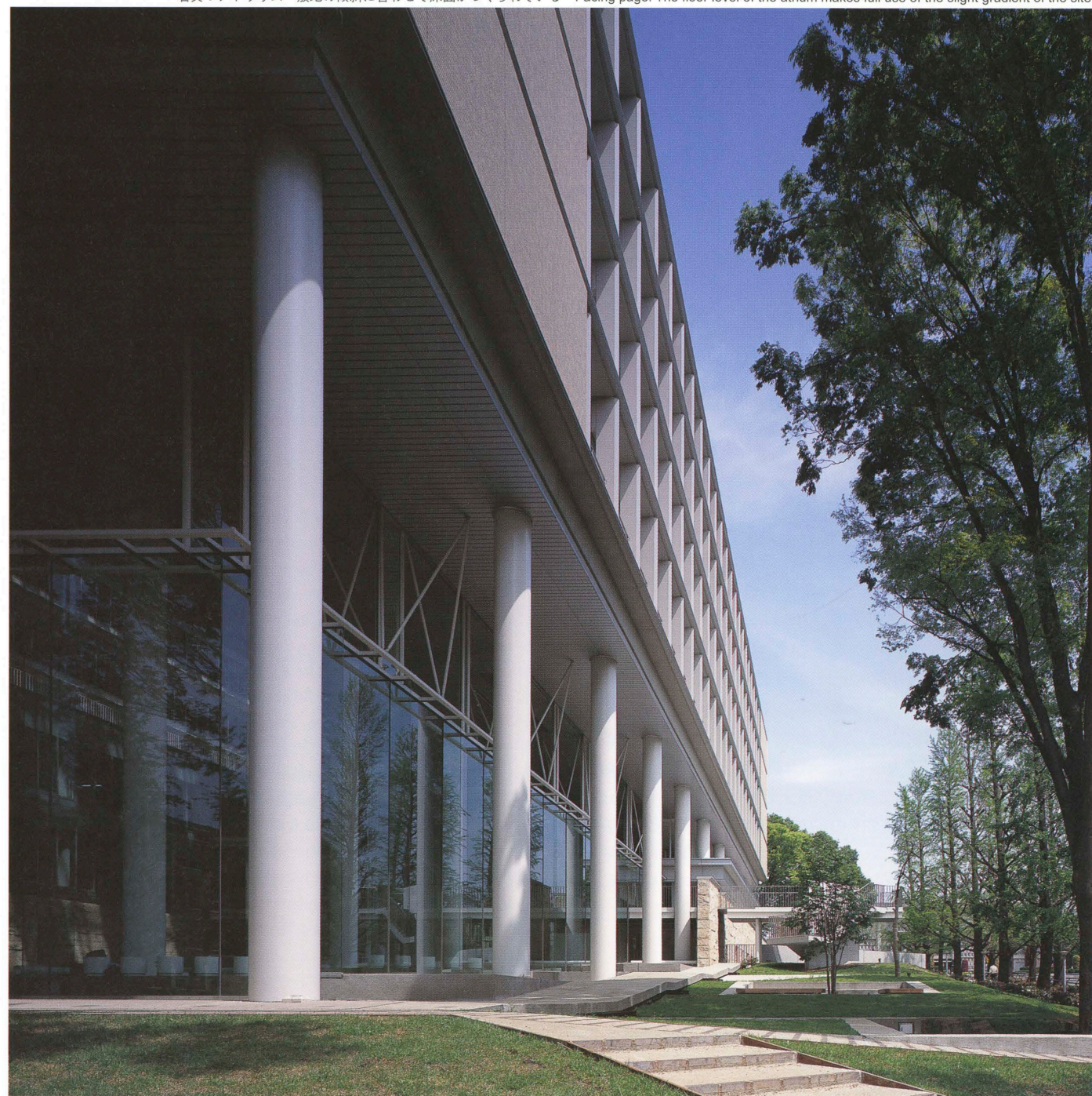
南側外観足元まわりを見る View of the foot of the building on the south side.
