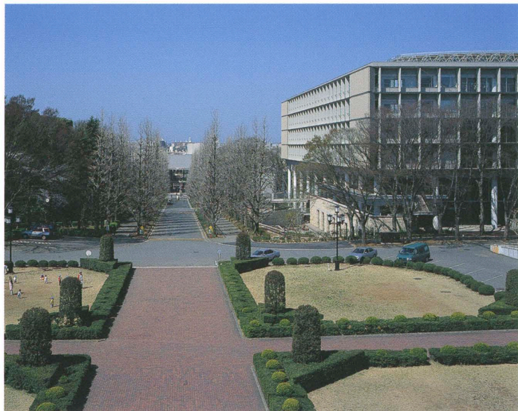
東側外観 中央がイチョウ並木 View from the east. Ginkgo trees lining the street.
