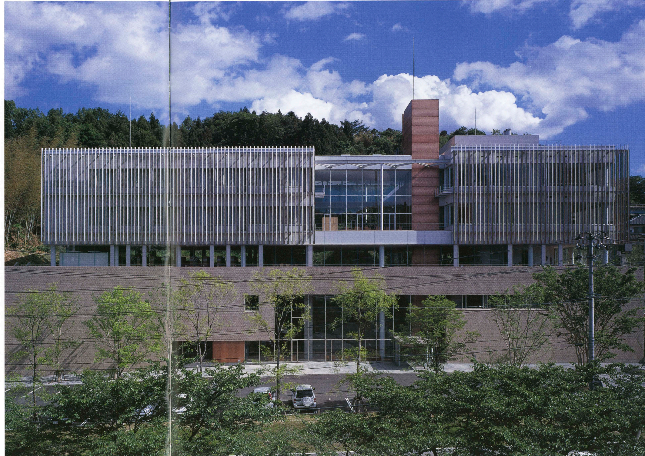
北側外観 Exterior on the north.
