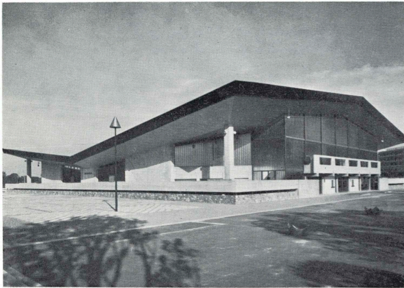
■ 屋内球技場西北面 Southern-north side of indoor ball court bldg.
