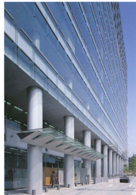
南玄関の東側外観 Southern entrance.
