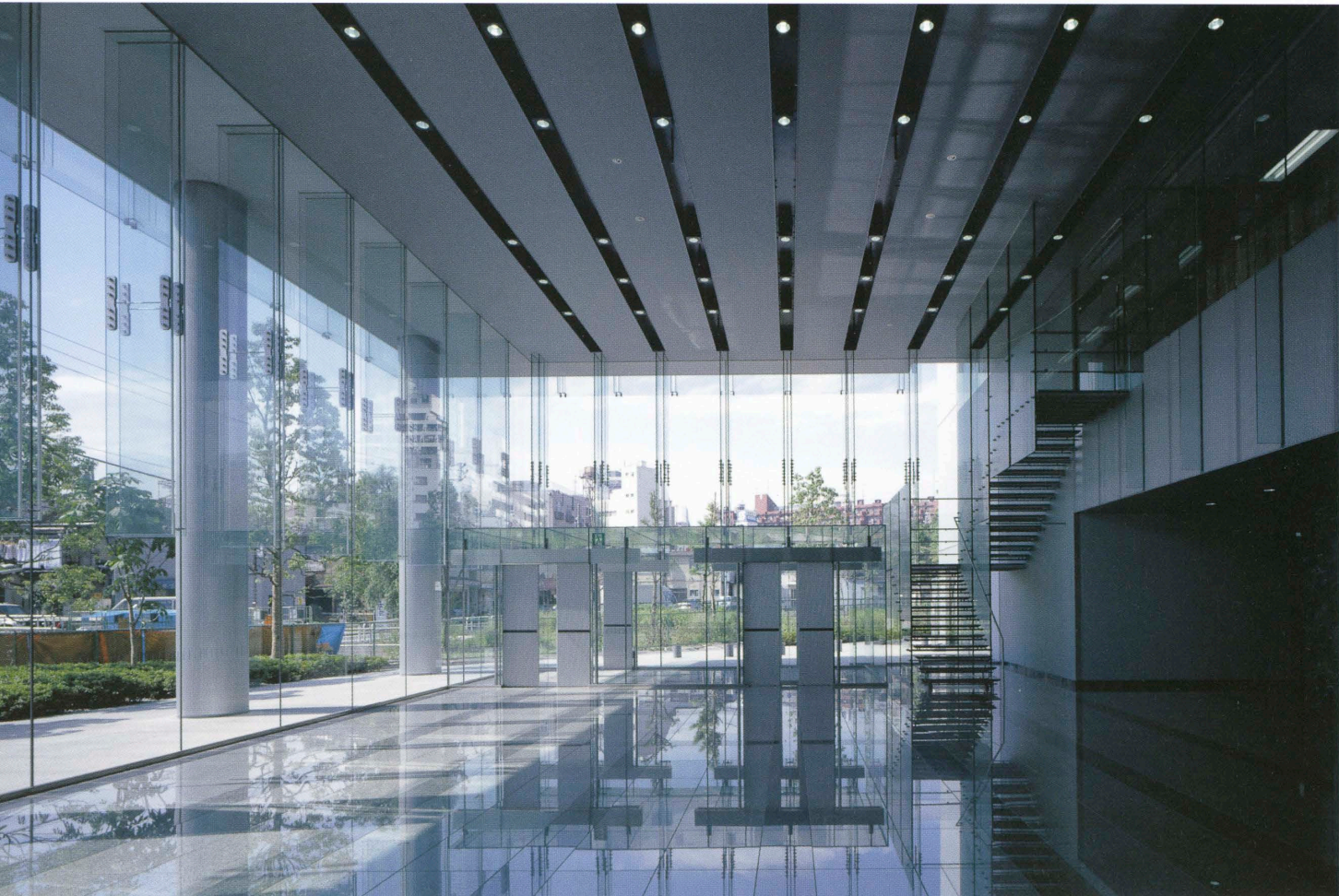
北玄関ホール北側を見通す Unobstructed view in the northern entrance hall.
