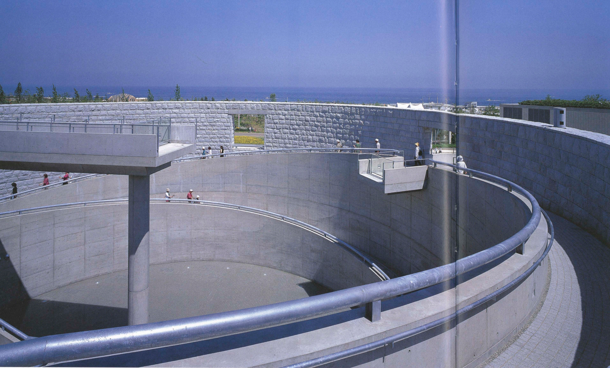
最高高さ約11mの石壁に囲まれた直径約32mの円形フォーラム Circular forum surrounding stone with a diameter of 32 meters and 11 meters high.
