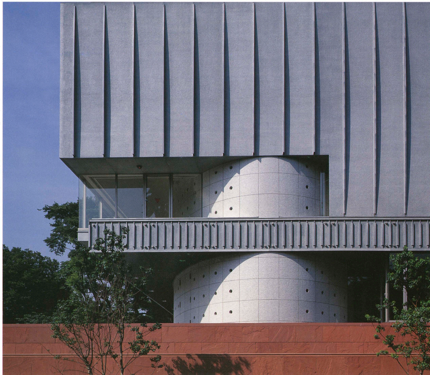
北側外壁の一部 Part of the exterior walls on the north.
