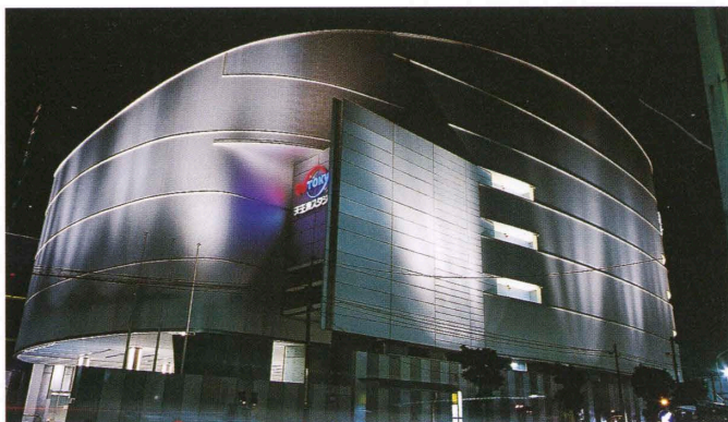
スタジオ棟夜景 Night view of the Studio wing.
