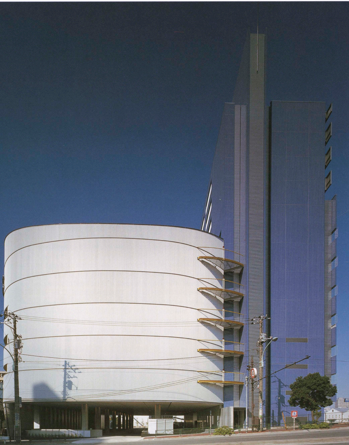
南側外観 低層部分がスタジオ棟、高層部分がオフィス棟 View from the south. Low-rise studio wing attached to the office tower.
