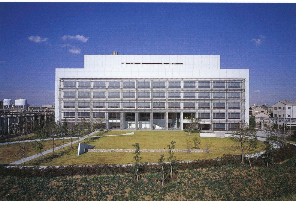
南側外観 General view from the south.
