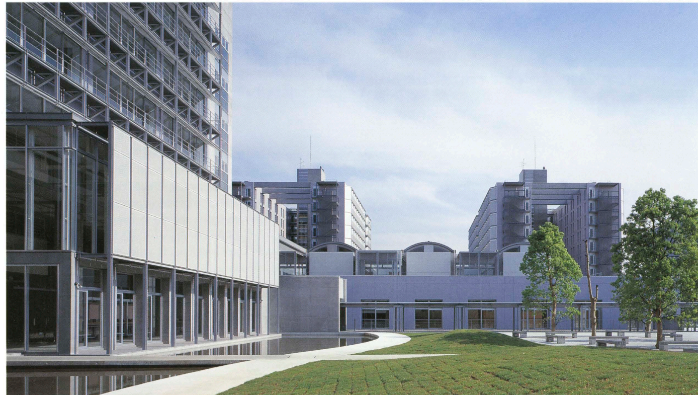
研修棟西側の池越しに南側を見る 正面手前が厚生棟、奥が学寮棟 View of the training building(left) and lowrised welfare building(front) facing the plaza.
