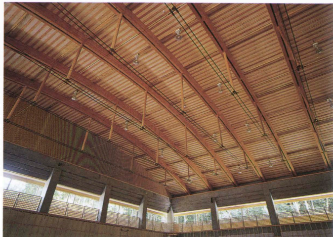
体育館見上げ Upward view of the gymnasium.
