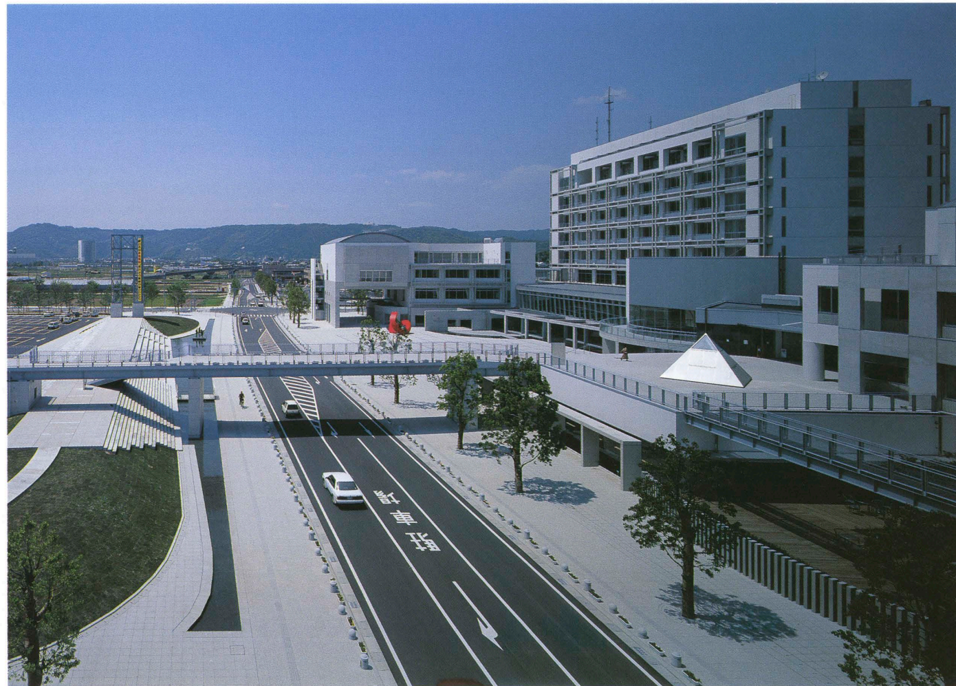
南東側全景 道路を挟んだ左はステージと駐車場 General view from the southeast. Stepped stage and parking area seen across the street on the left.
