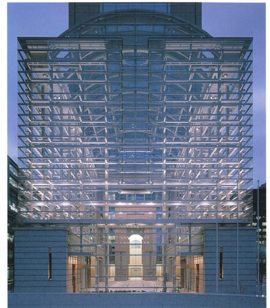
屋内公開空地のアトリウムタ景 Twilight view of the atrium which is also the public open space.
