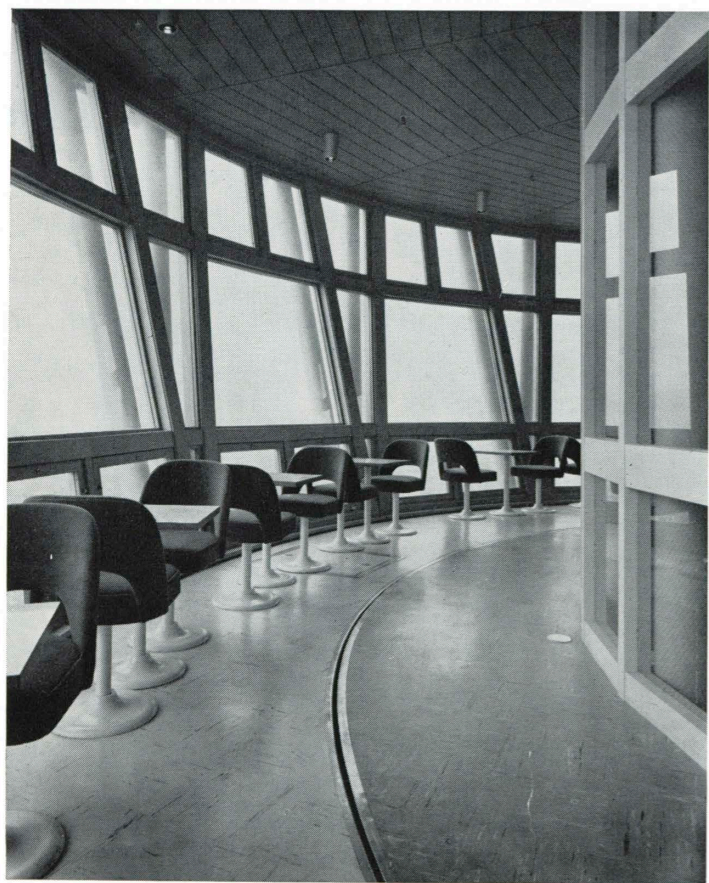
■ 展望階 3 階喫茶室内部回転床 tea room rotating floor-3rd observation floor
