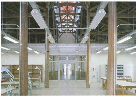
既存倉庫を改修した実習室 Practical training room remodeled from the existing storage.
