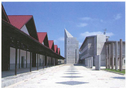
南側外観 外路は貨物引込み線が走っていた Southward view. Pavement reconstructed on the sidetrack of the freight.
