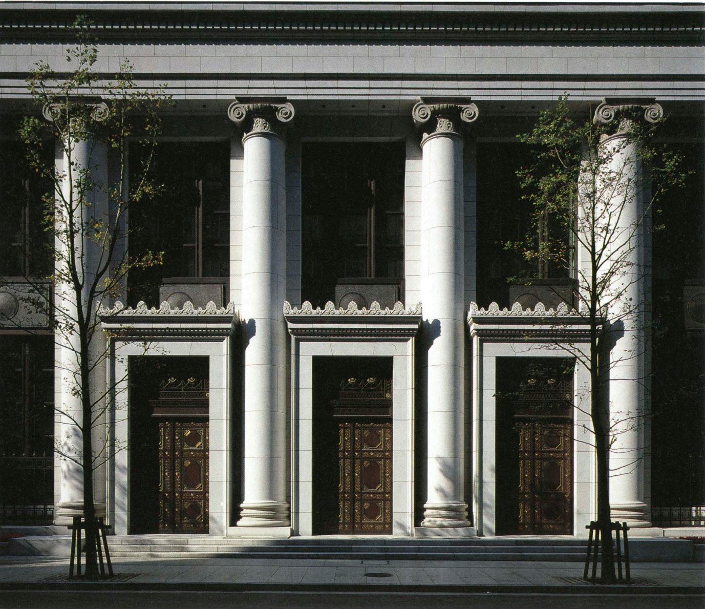
低層部東側外観 Eastern exterior preserving some part of the existing building.
