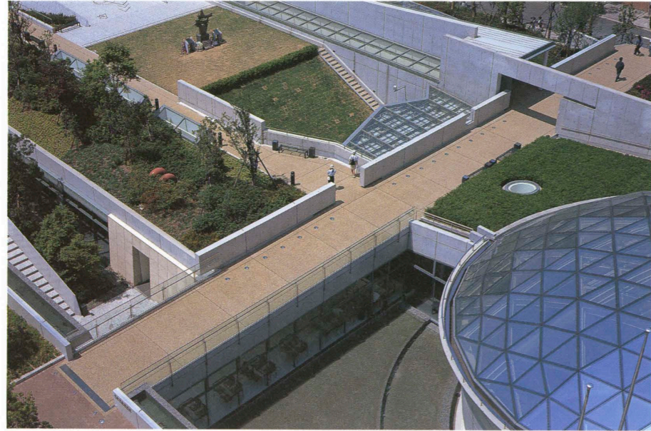
平和会館側アプローチ見下ろし Downward view of the paved approach on the rooftop from the east of the park.
