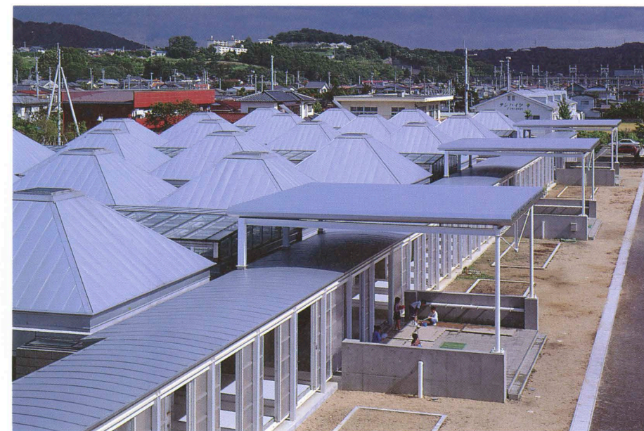
教室ゾーン屋根の並び The sequence of roof forms in the classroom zone.
