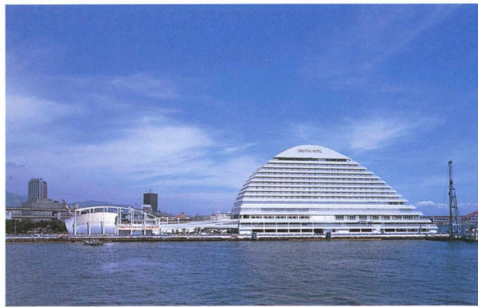
西側全景 General view from the west.
