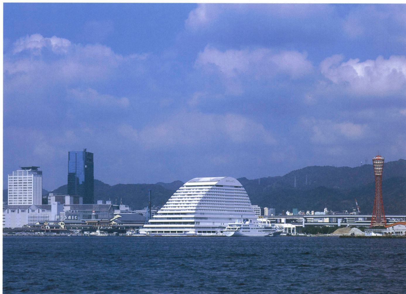
南東側遠景 Distant view from the southeast.
