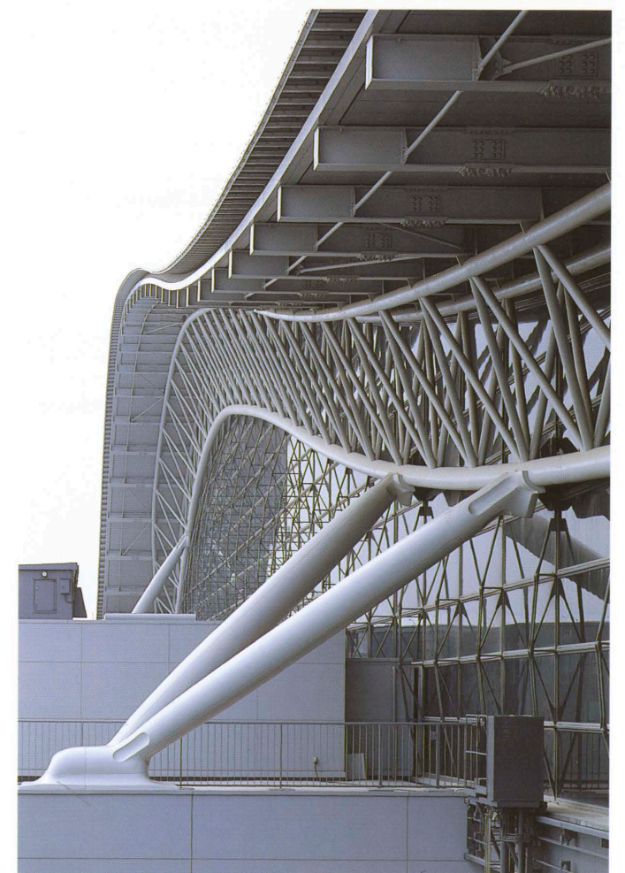
MTB妻側 Gable end of the Main Terminal Building(MTB).
