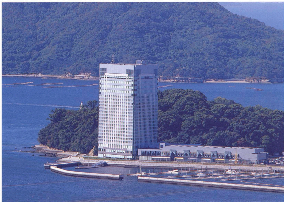
北東からの遠望 Distant view from the northeast.
