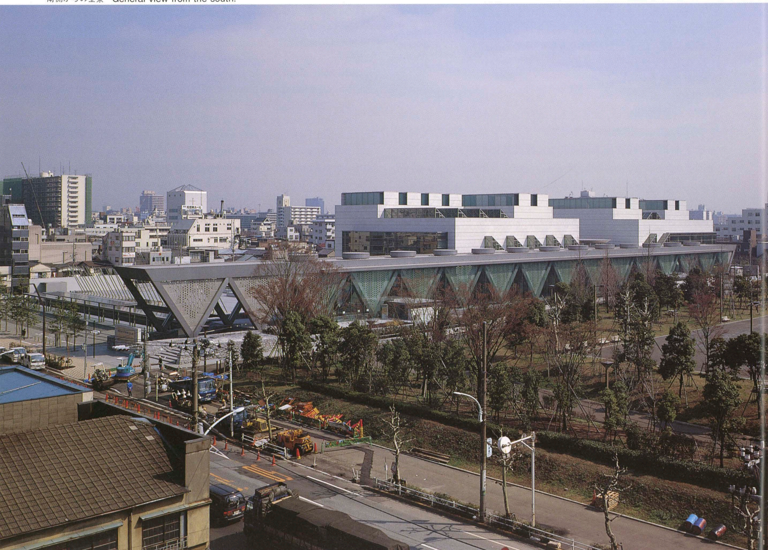
南側からの全景 General view from the south.
