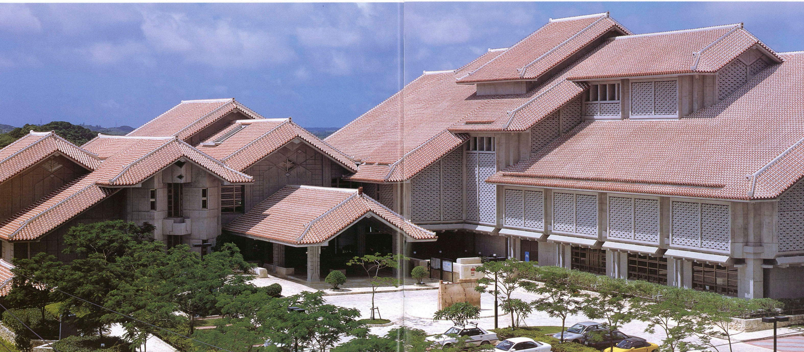
北より見る、屋根は沖縄産瓦本葺き View from the north. The roof is covered with traditional Okinawa tiles.
