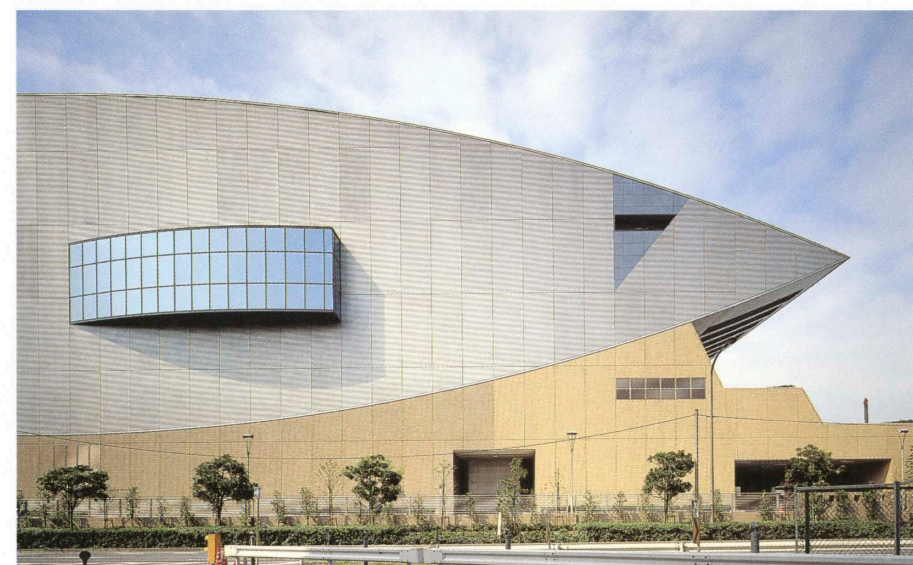
南側壁面 Exterior on the south.
