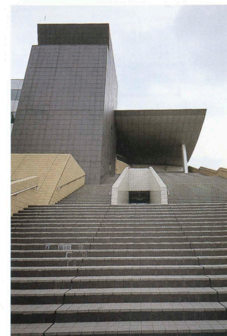
階段見上げ Upward view of the stairs.
