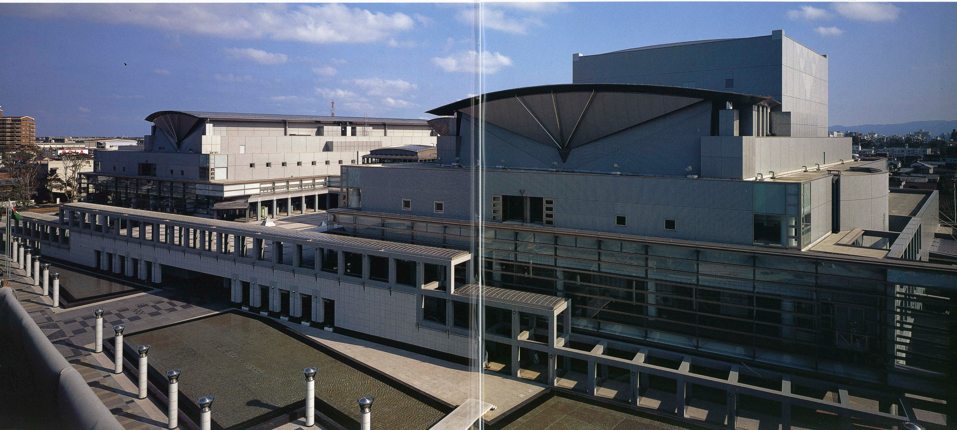
南東側外観 General view from the southeast.
