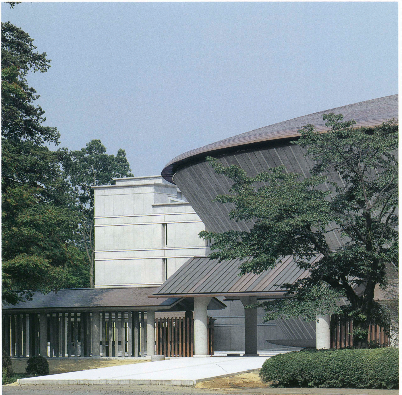
西側より回廊の正門越しに納骨堂を見る Inverted cone-shaped ossuary seen over the main gate and colonnade.
