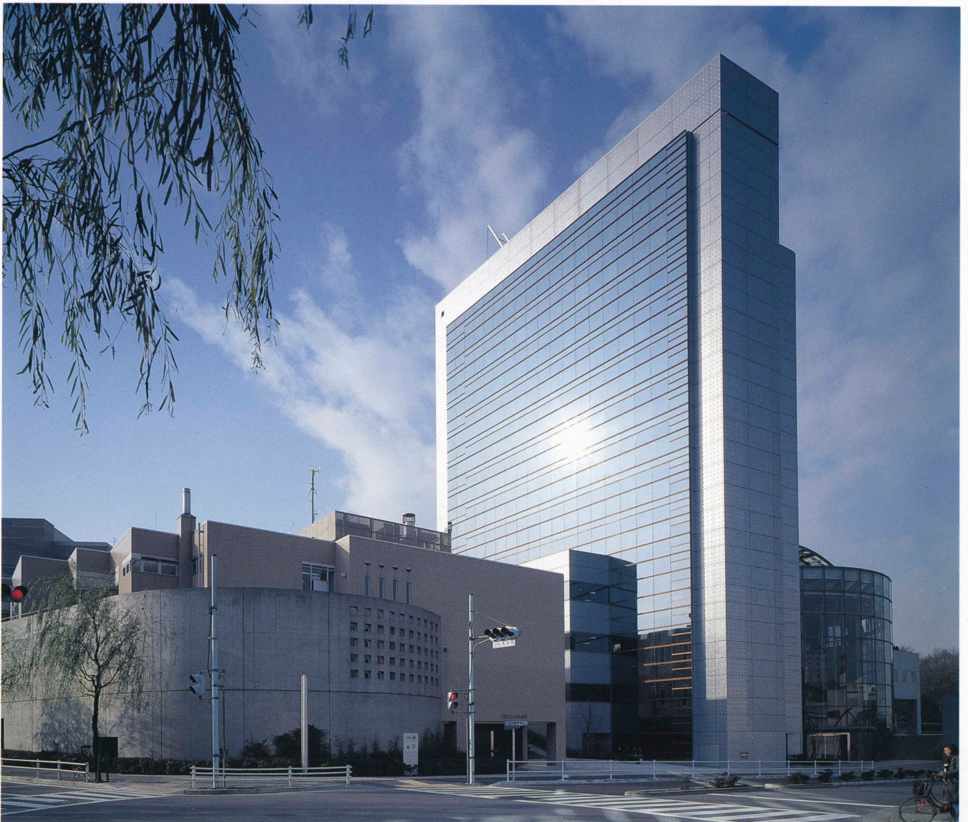
南東側外観 View from the southeast.
