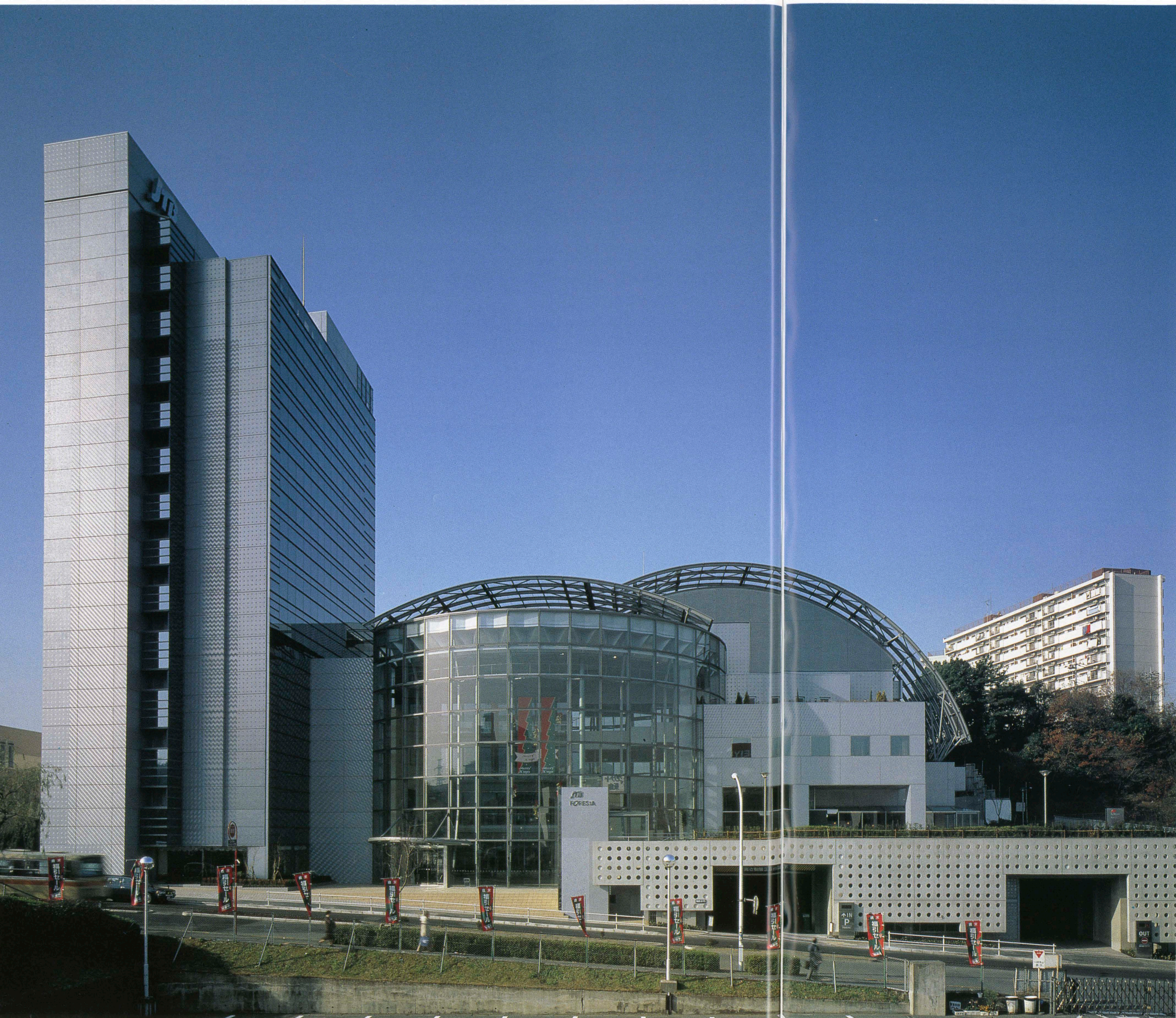
東側外観 Facade on the east.
