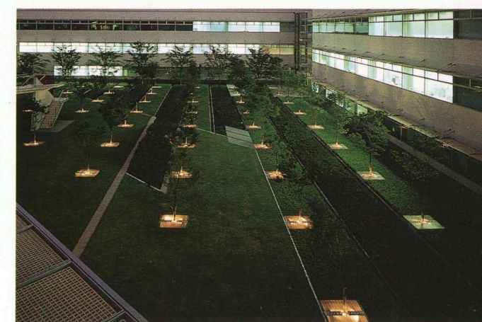
中庭夜景 Night view of the inner court.
