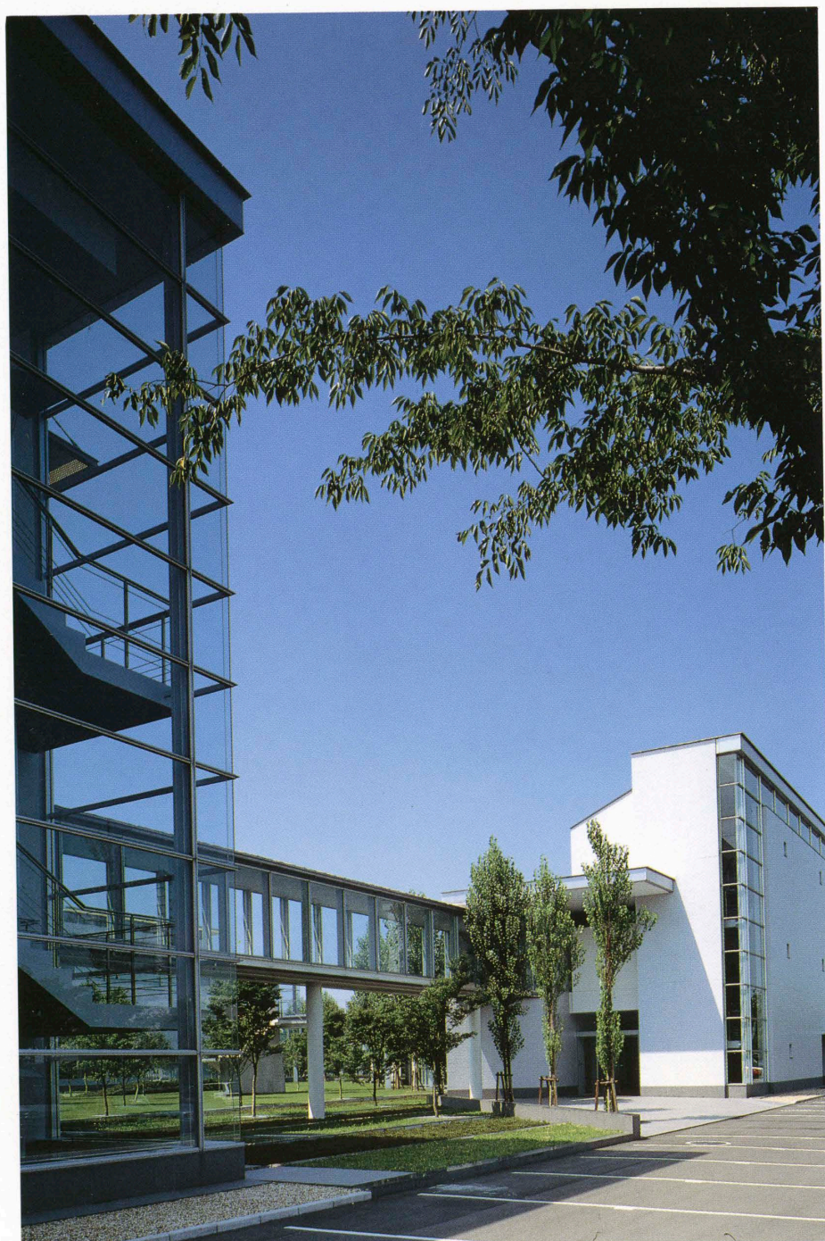
C棟側より渡り廊下とA棟を見る Overpass and A-wing seen from the northeast.
