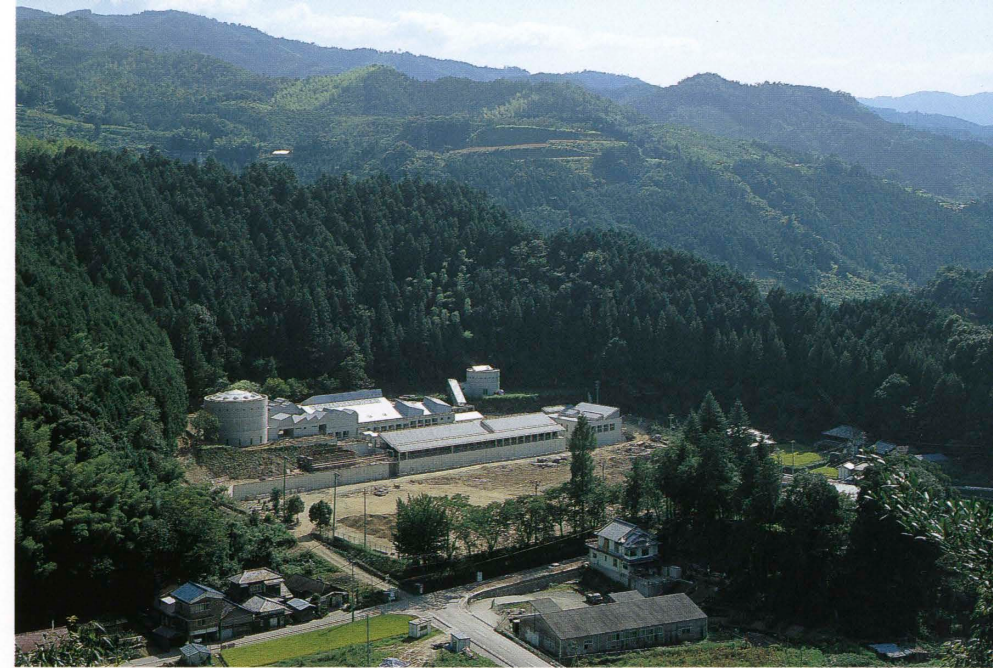
北東より全景 General view from the northeast.
