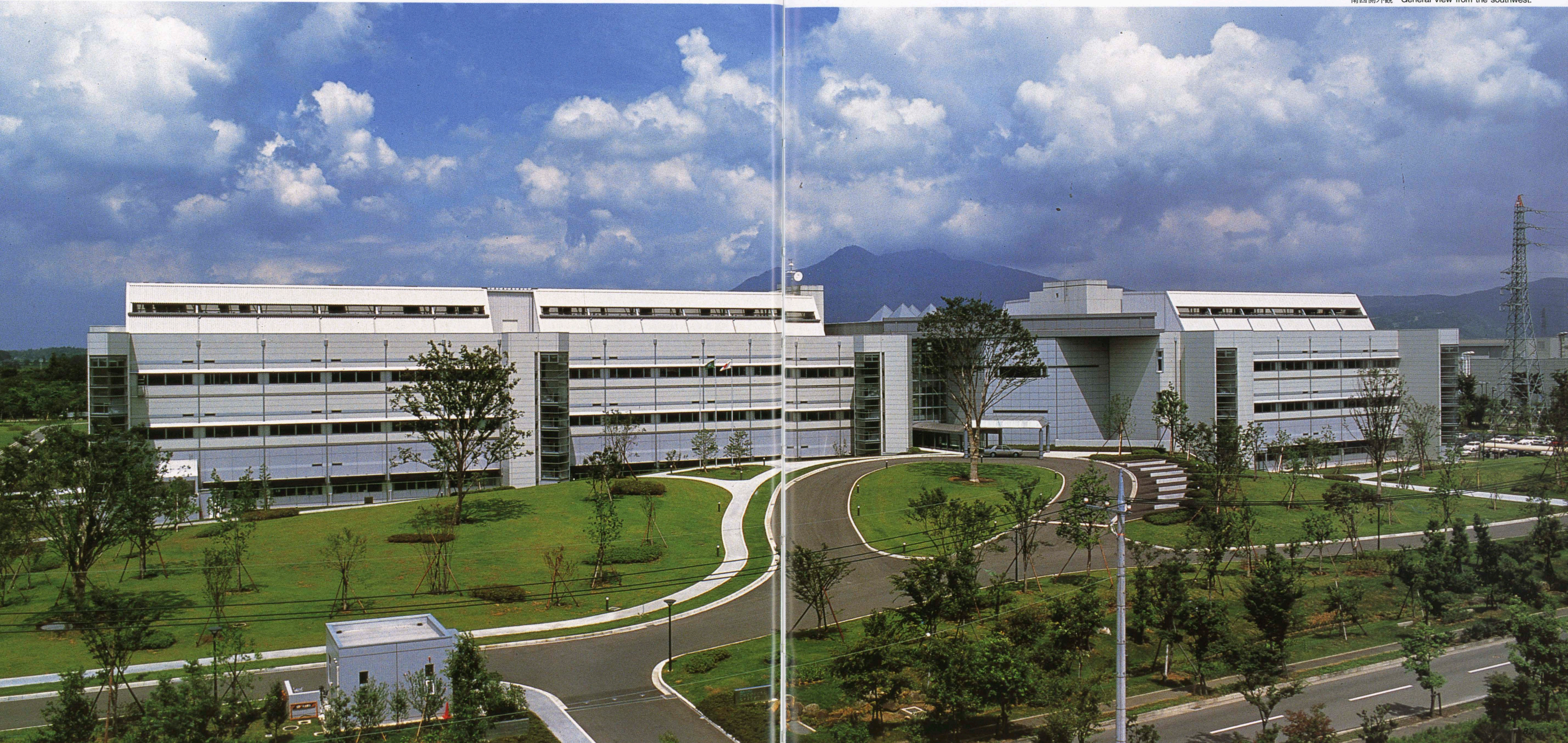
南西側外観 General view from the southwest.
