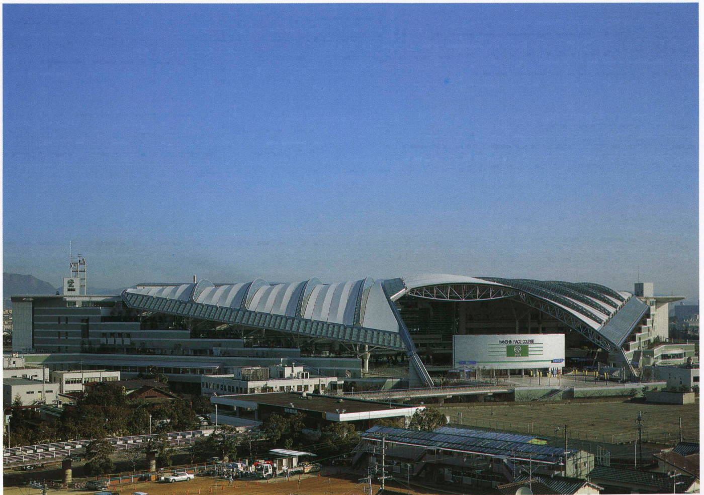
南西側全景 General view from the southwest.
