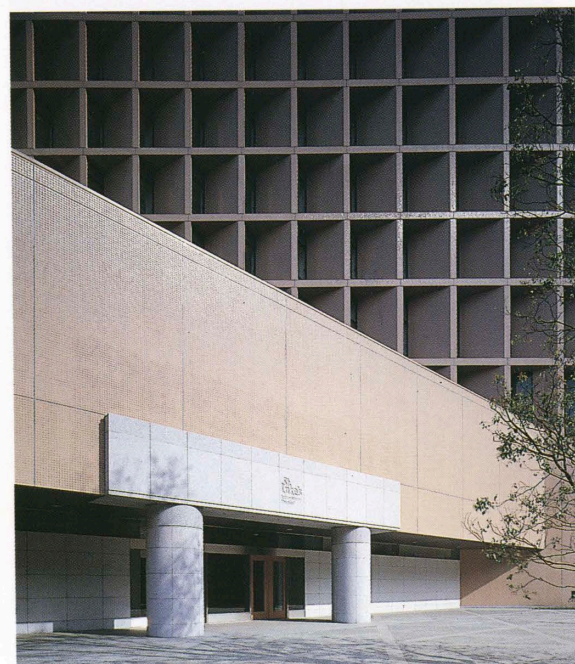
西側歩行者用玄関 Entrance for the foot-passengers.
