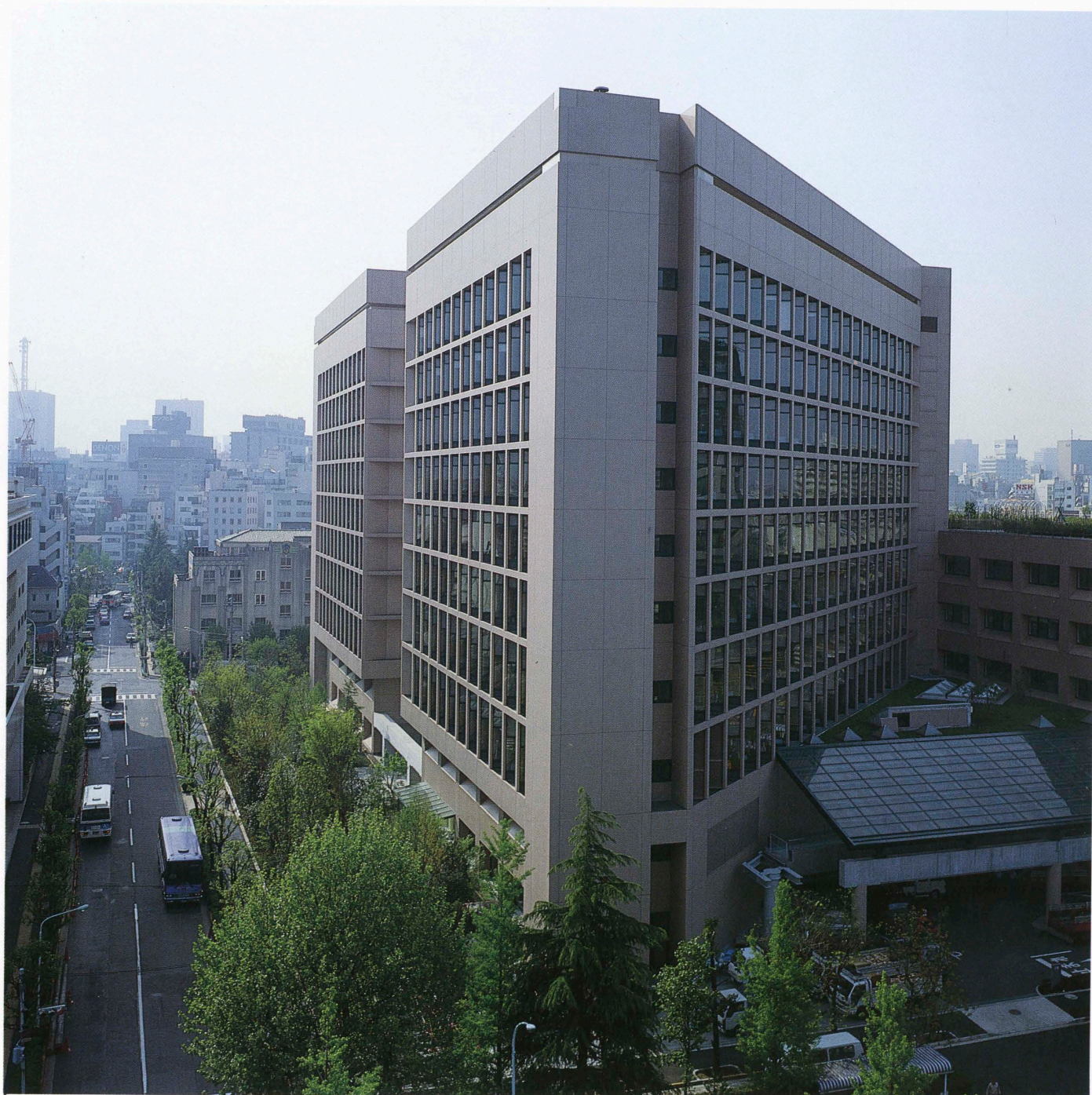
南東側外観 General view from the southeast.
