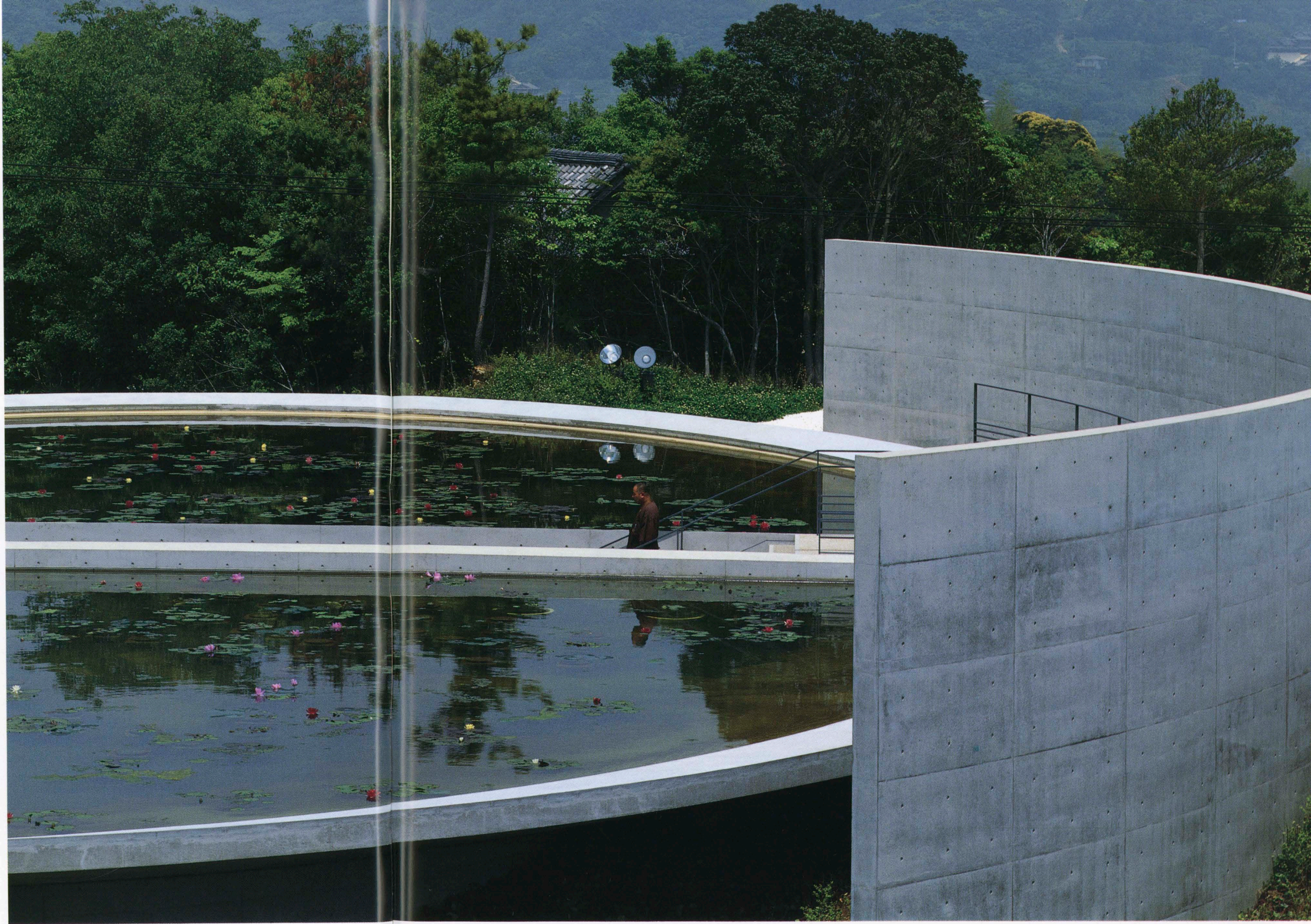
南西側より蓮池を見る Pond of lotus viewed from the southwest.
