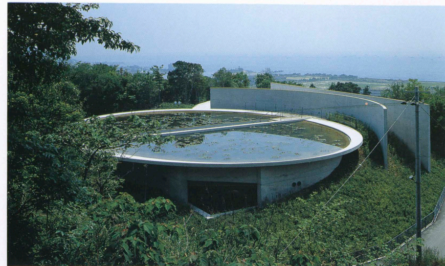
西側全景 General view from the west.
