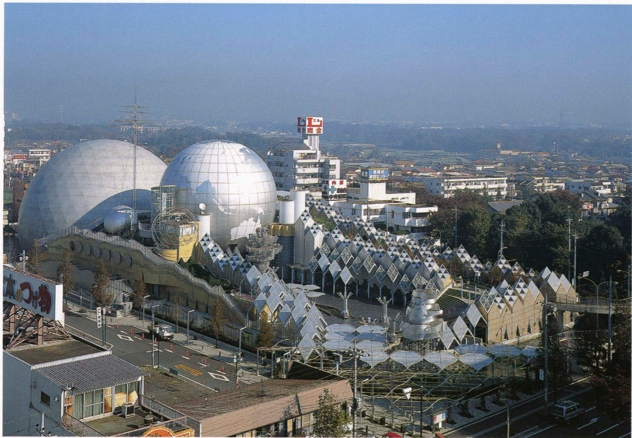
南西よりの全景 General view from the southwest.
