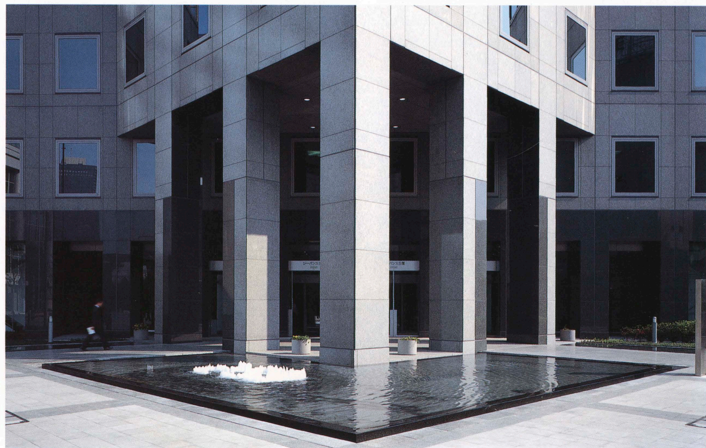
S館北側玄関回り Main entrance of the S-Building.
